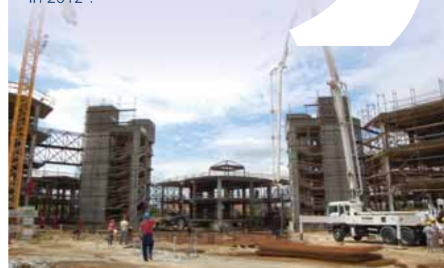
Zvezdara Technology Park under construction
